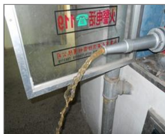
Photo of the inside of the main production hall Hydrant test.JPG
